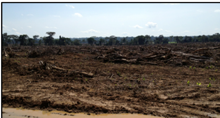
Land Clearing at ATAMA Plantation for oil palm (April 2013)
